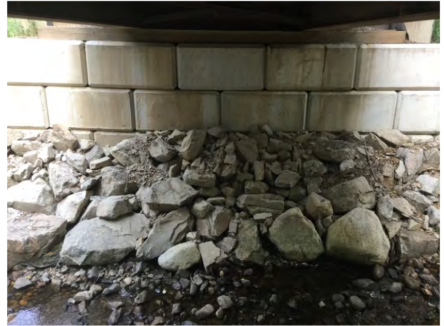
Right Bank Abutment when facing downstream
