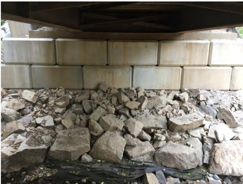
Left Bank Abutment when facing downstream
